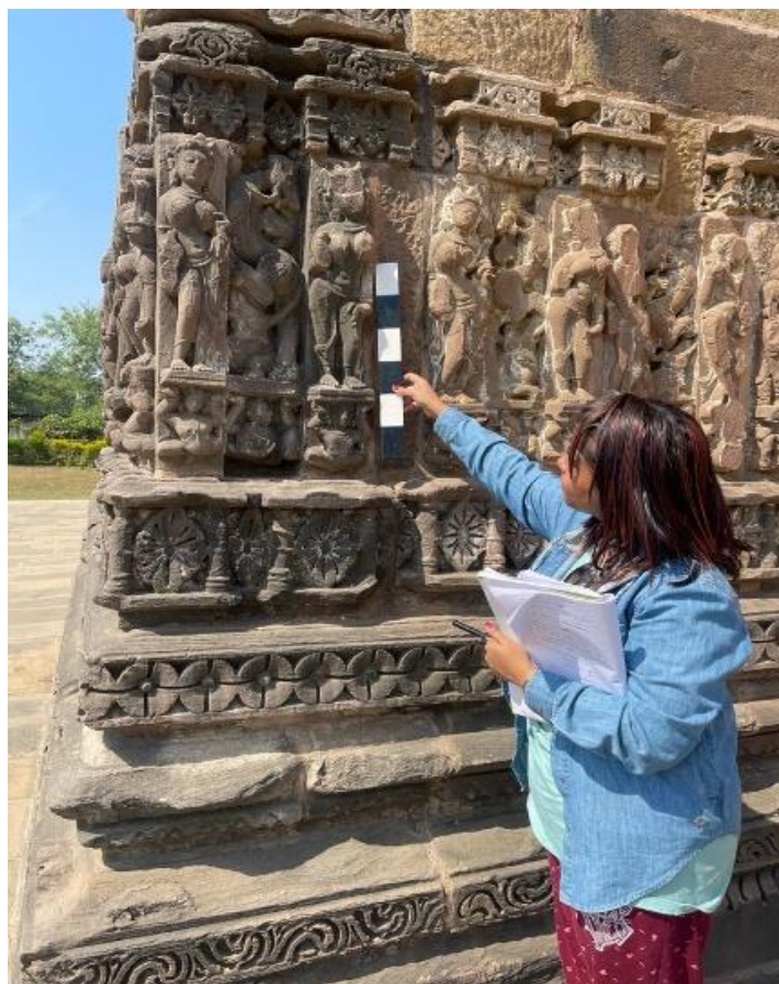
Figure 6 The Outer Wall Of The Temple
